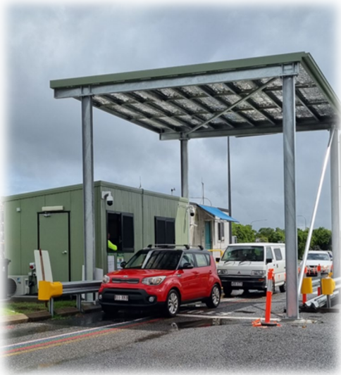
The new gatehouse in place
